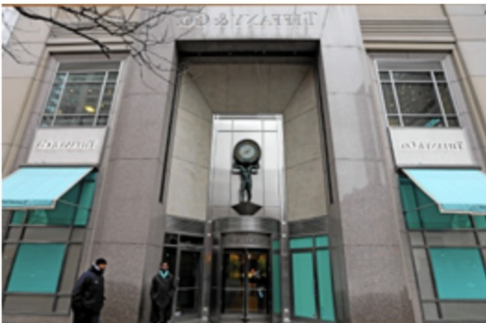
Complete renovation of New York City flagship store
