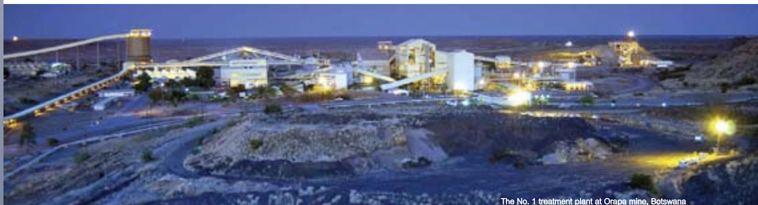
The No. 1 treatment plant at Orapa mine, Botswana
